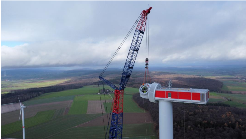
Construction of the new wind turbine
