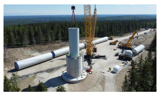
PHOTO: The foundations of the Lumivaara turbines have been raised to take advantage of the stronger winds blowing at higher altitudes and to maximise energy production from the turbines, which means that the climate impact of the additional concrete used in the foundations will be compensated in just a few years.
