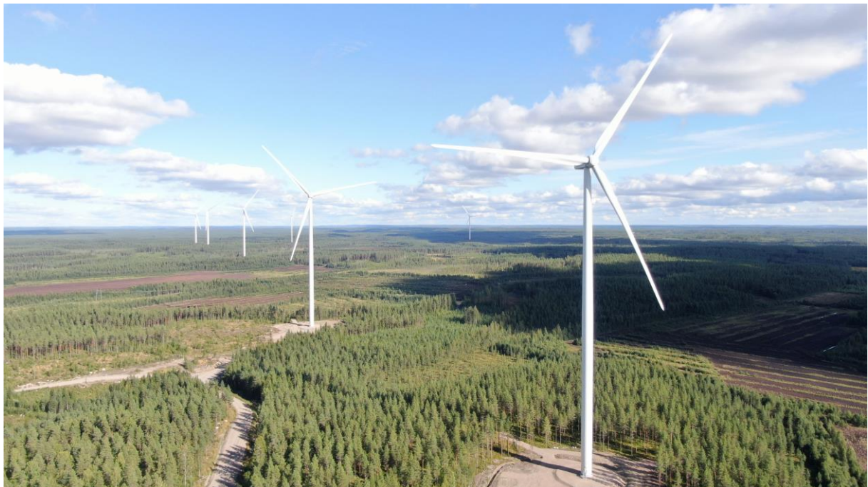
Photo: The Konttisuo wind farm in Finland went online in 2022 and contributed to the company's success.
