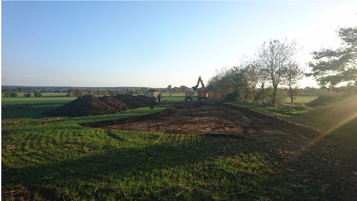
Photo: St. Morand construction site
